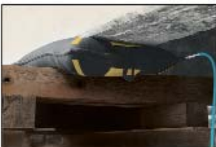
Lifting a bridge. That's right; a bridge.
