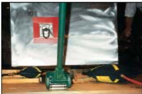
Raise loads to place industrial rollers.
